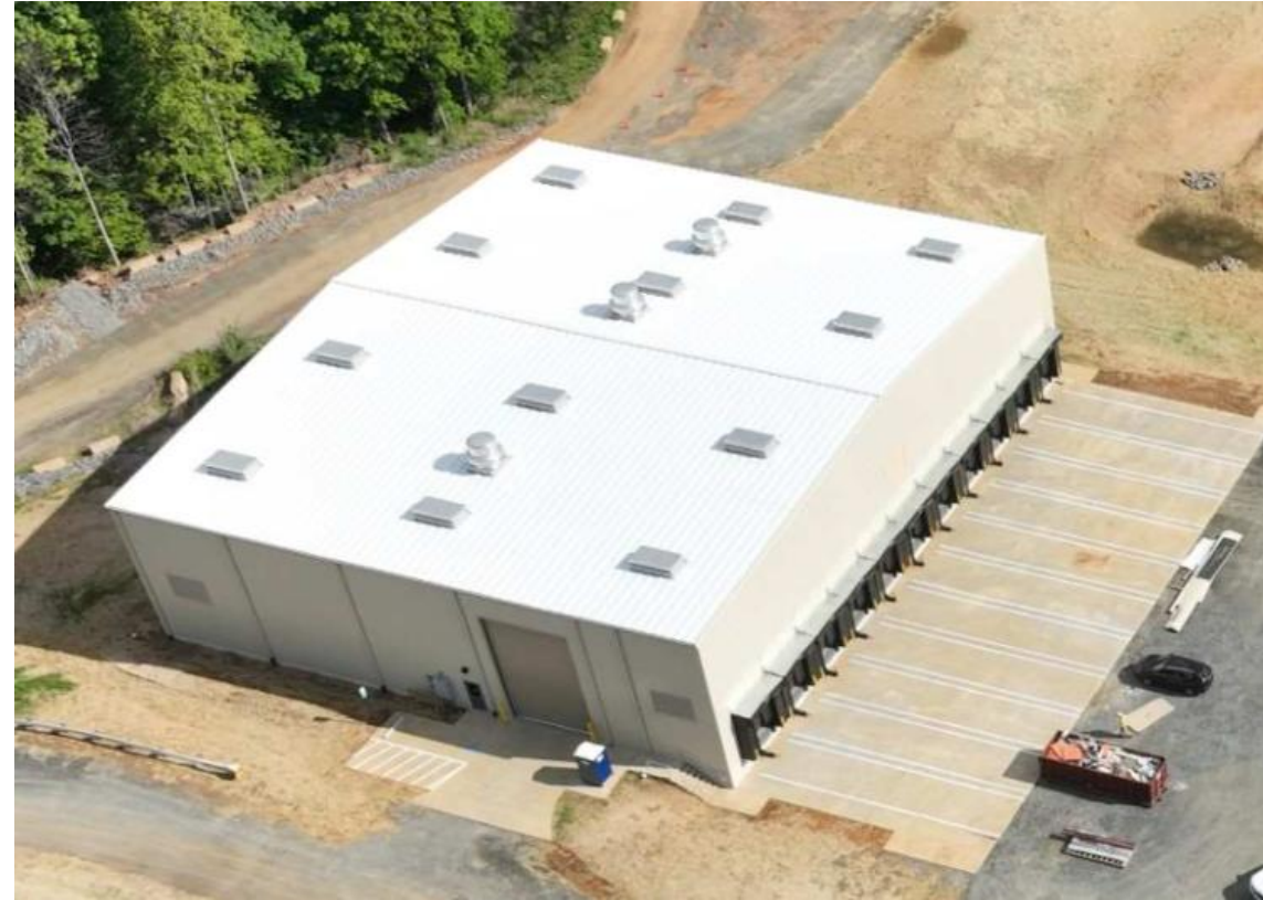
Baling Facility at end of construction
