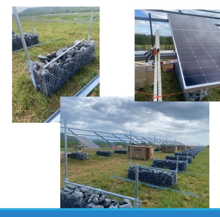
Gabion boxes: wire mesh containers filled with rock, are used for civil engineering applications. In this solar project, they are used as structural supports for the solar panels.
